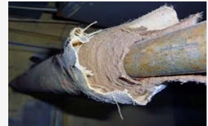
Grease duct gasket, pipe "lagging" and insulation containing asbestos
