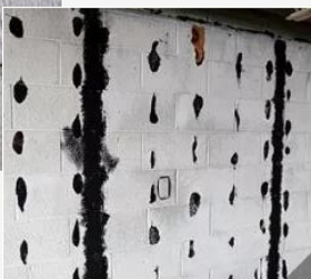
Ceiling tile pucks and wall adhesive containing asbestos
