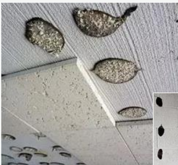
Ceiling tile pucks and wall adhesive containing asbestos
