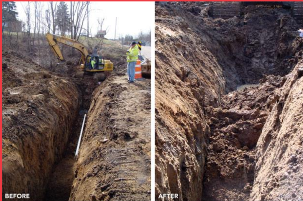
On March 8, an OSHA inspector ordered a worker out of a trench at a construction site in Mercerville, OH, (above, left) minutes before a portion collapsed (above, right).
