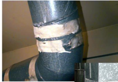
SEAM TAPE ON FURNACE DUCT (BOAT WORKS, HOPKINS MARINE STATION)
