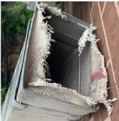
ASBESTOS CLOTH AT EXHAUST DUCT & FAN CONNECTION (HERRIN LAB)
