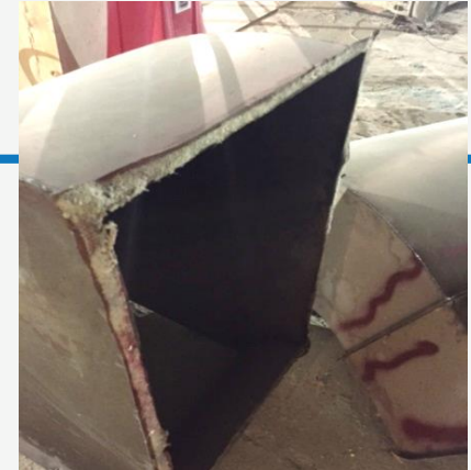
Grease duct gasket, pipe "lagging" and insulation containing asbestos
