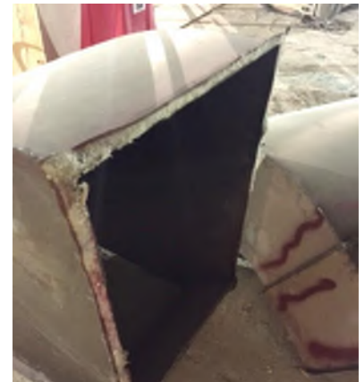
Grease duct gasket, pipe "lagging" and insulation containing asbestos
