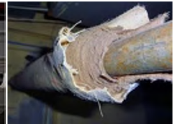
Grease duct gasket, pipe "lagging" and insulation containing asbestos
