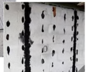
Ceiling tile pucks and wall adhesive containing asbestos
